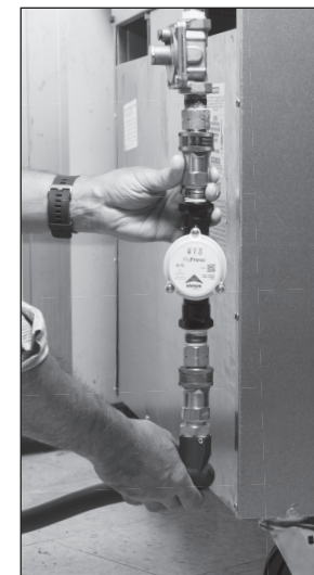
Fig. C Gas Range outfitted with the new FloPro-MD with QD Kit.
