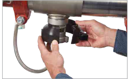
2. Position the two halves of the sensor on the relief valve.
